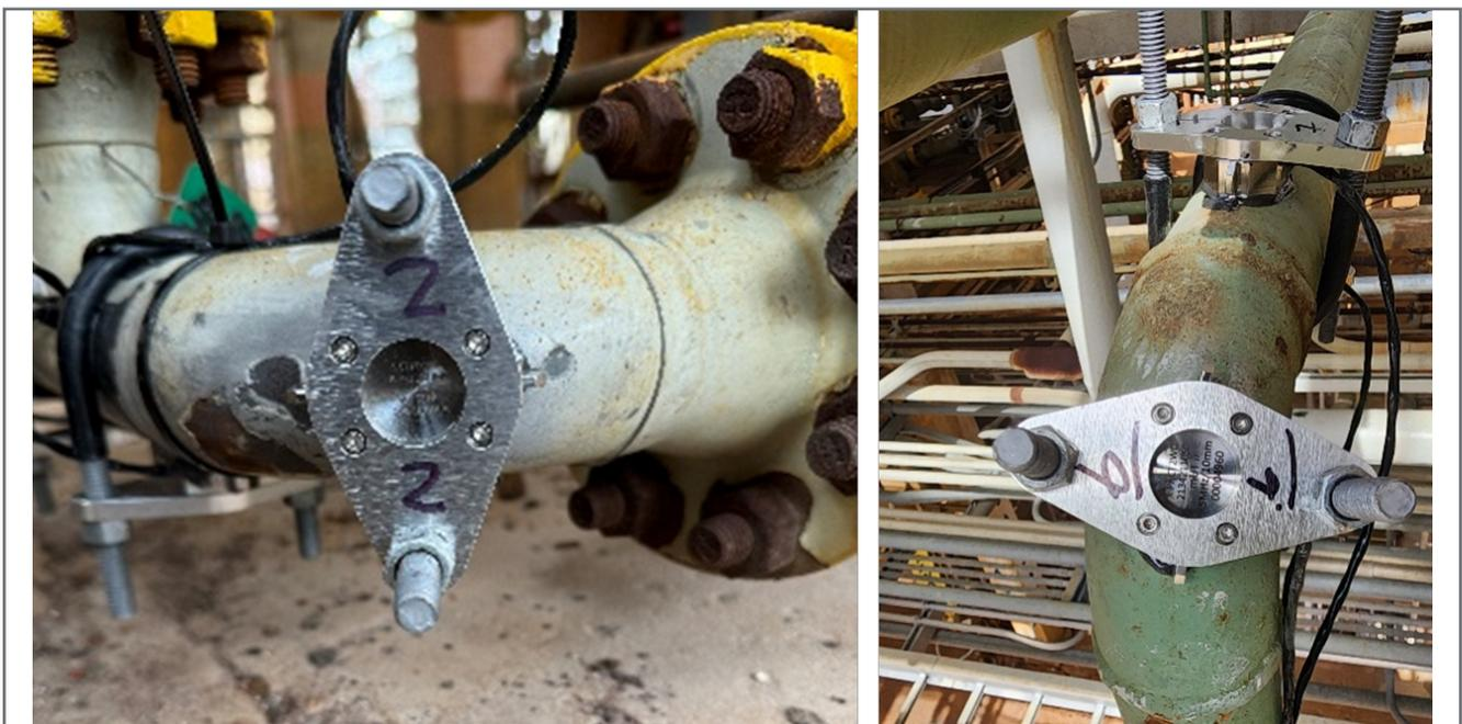
Figure 1: Ultrasonic Sensors with Mounting Fixtures on 2-inch Piping
